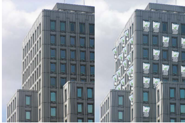
Figure 4. Incorporating greenery into building, before and after.
