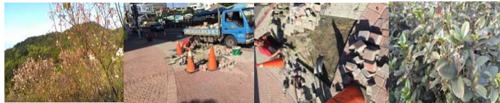
Figure 7. Taipei's Chunghsiao Road, new North road pavement
