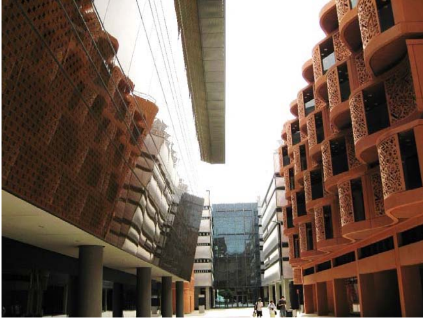
Figure 2. Contemporary screens Masdar City
